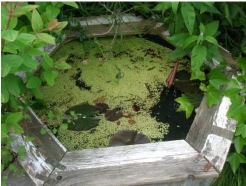
4.9 The living machine uses vegetation to treat waste water. Photo by Bruce Haglund.
