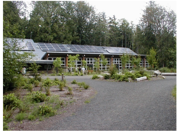
4.2 Photovoltaic arrays on the building roofs help to power IslandWood. Photo by Bruce Haglund.
