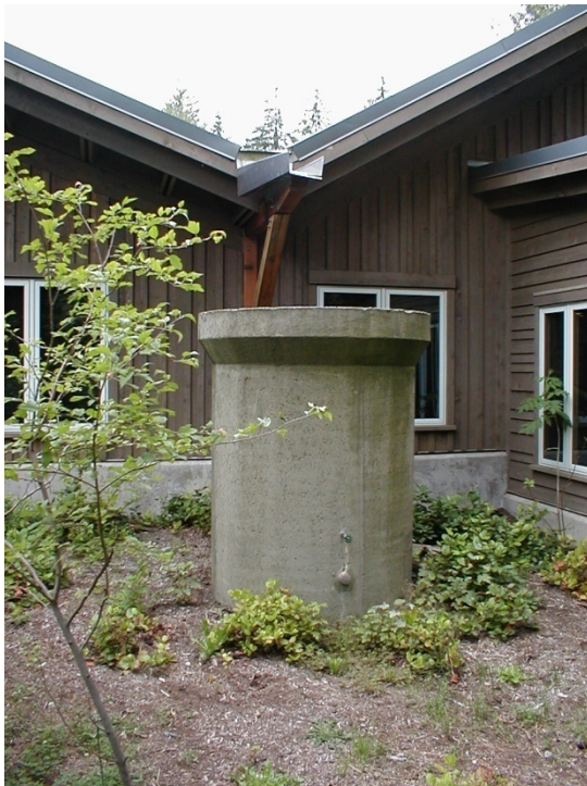
4.5 The butterfly roofs drain rainwater into cisterns for water storage. Photo by Bruce Haglund.
